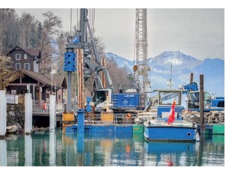
The Swiss company Kibag is installing new mooring piles for the Lake Lucerne Navigation Company. For the first time, Kibag is using a drilling rig from Liebherr's LB series. The LB 30 is facing challenges which literally couldn't be
