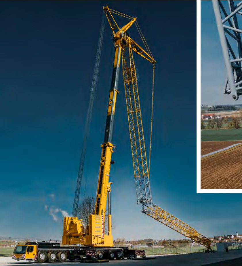
Erect the luffing jib in two parts - Redressement de la pointe basculante en deux parties
