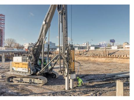
The piling rig LRH 100.1 unplugged is one of the latest models in the electrically driven unplugged series from Liebherr. Fitted with a hammer H 6, it has found its first jobsite in Sweden.
