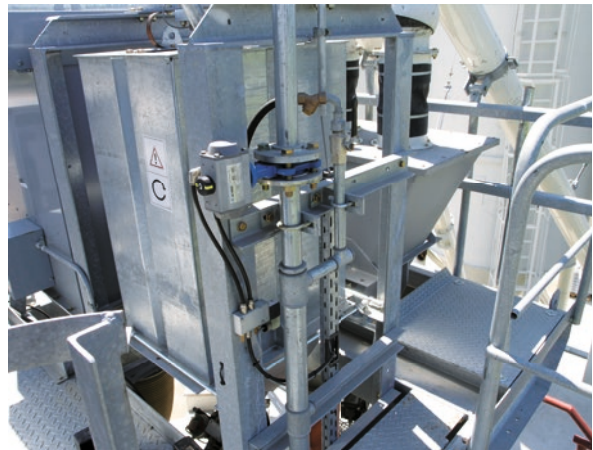
The large-scale weighing platform, with cement and water weighers, has good maintenance access.
