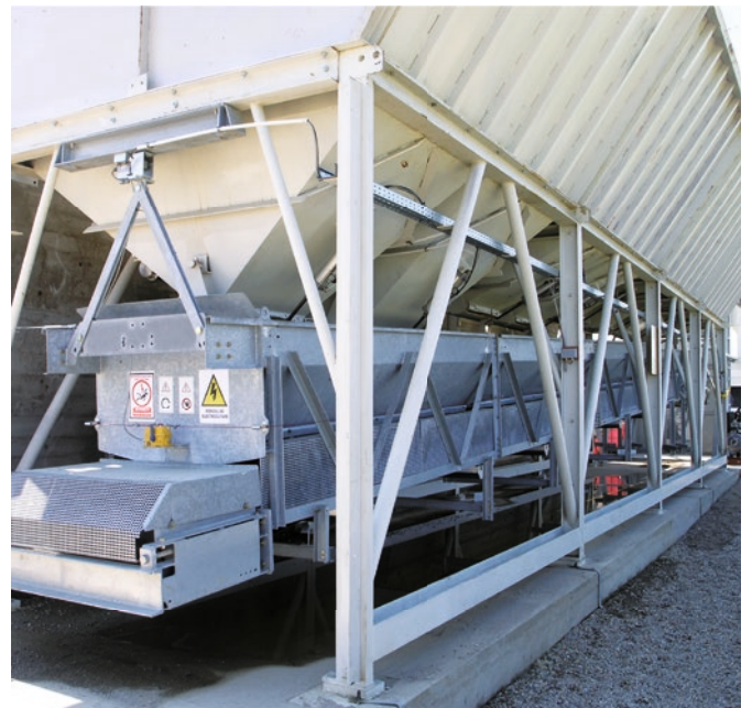
The belt weigher beneath the in-line silo.
