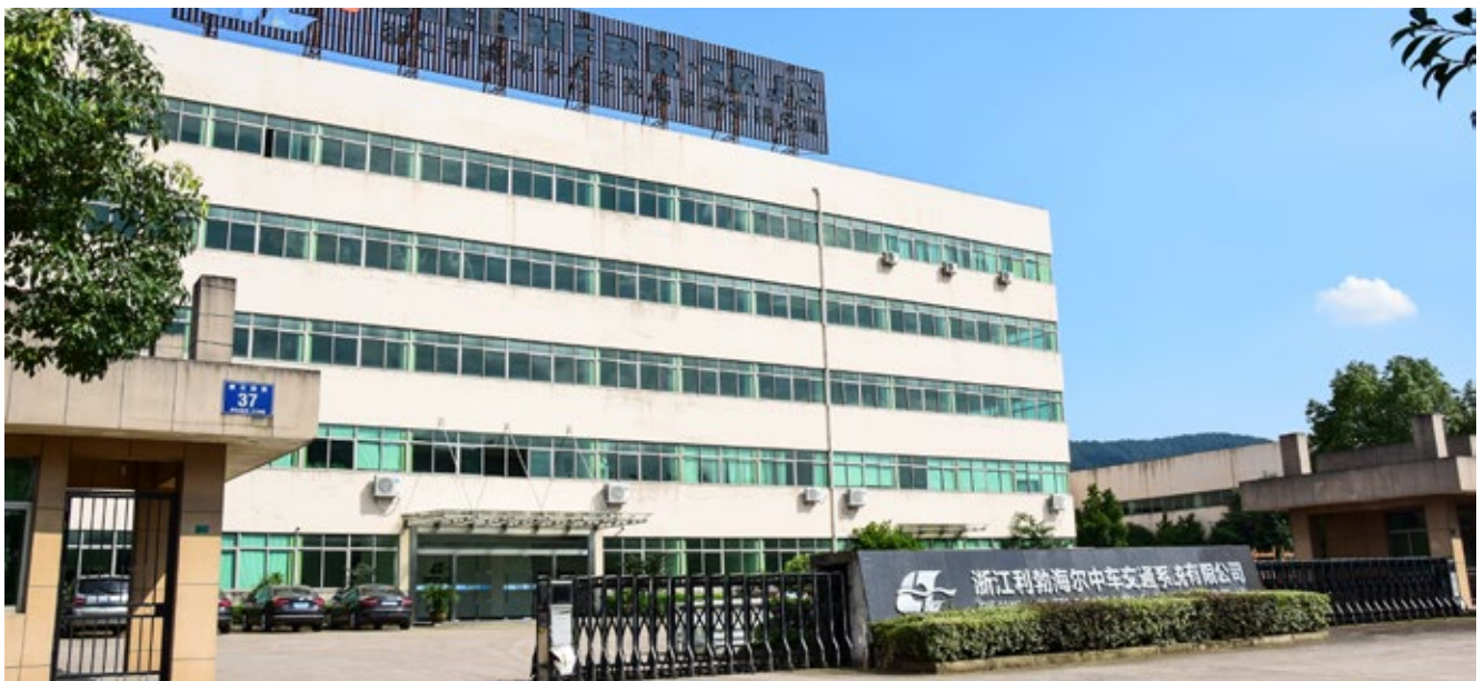
Zhejiang Liebherr Zhongche Transportation Systems Co., Ltd. in Zhuji
