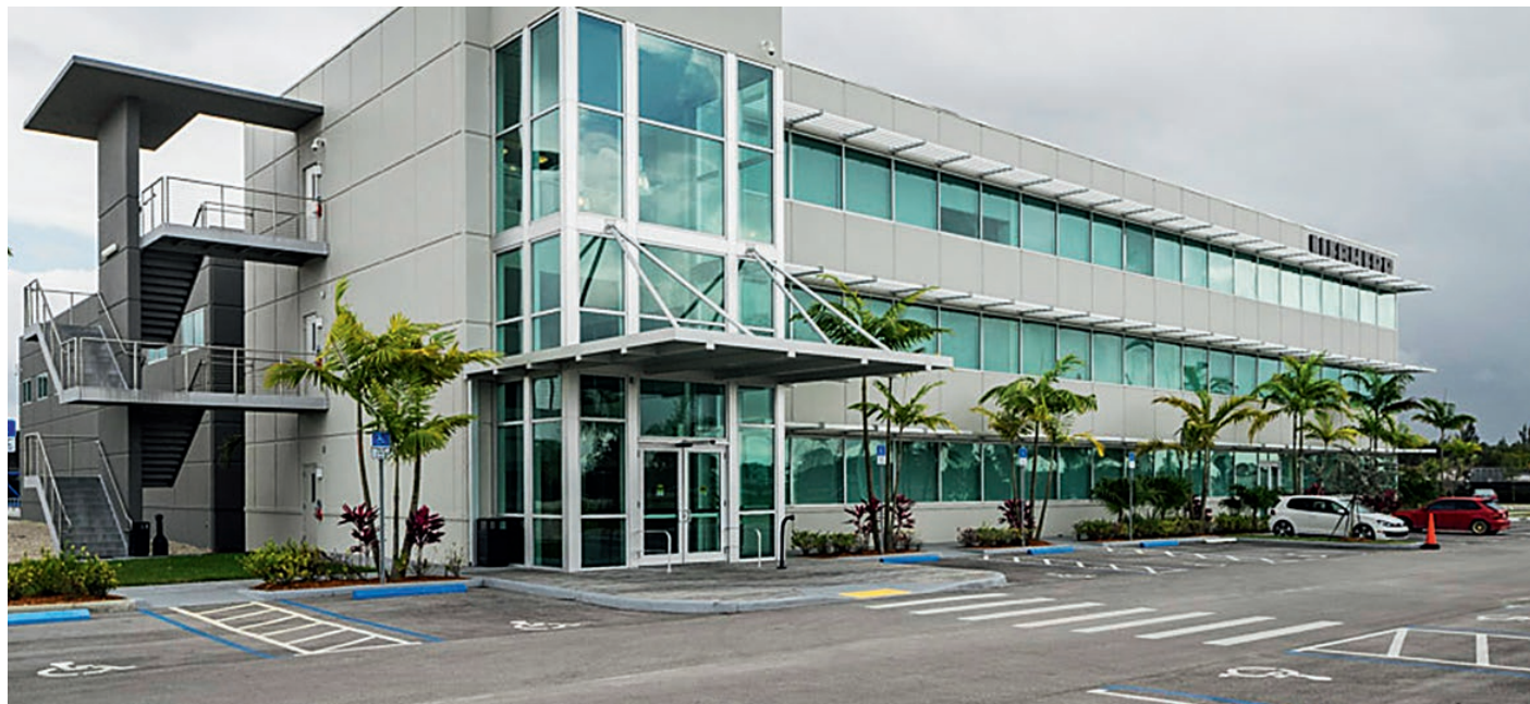
Liebherr offices in Miami, Florida, USA
