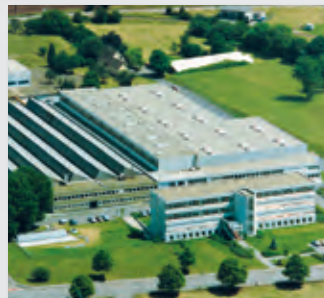
Ettlingen (Germany): remanufactured components
