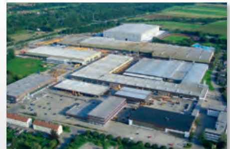
Kirchdorf (Germany): hydraulic cylinders
