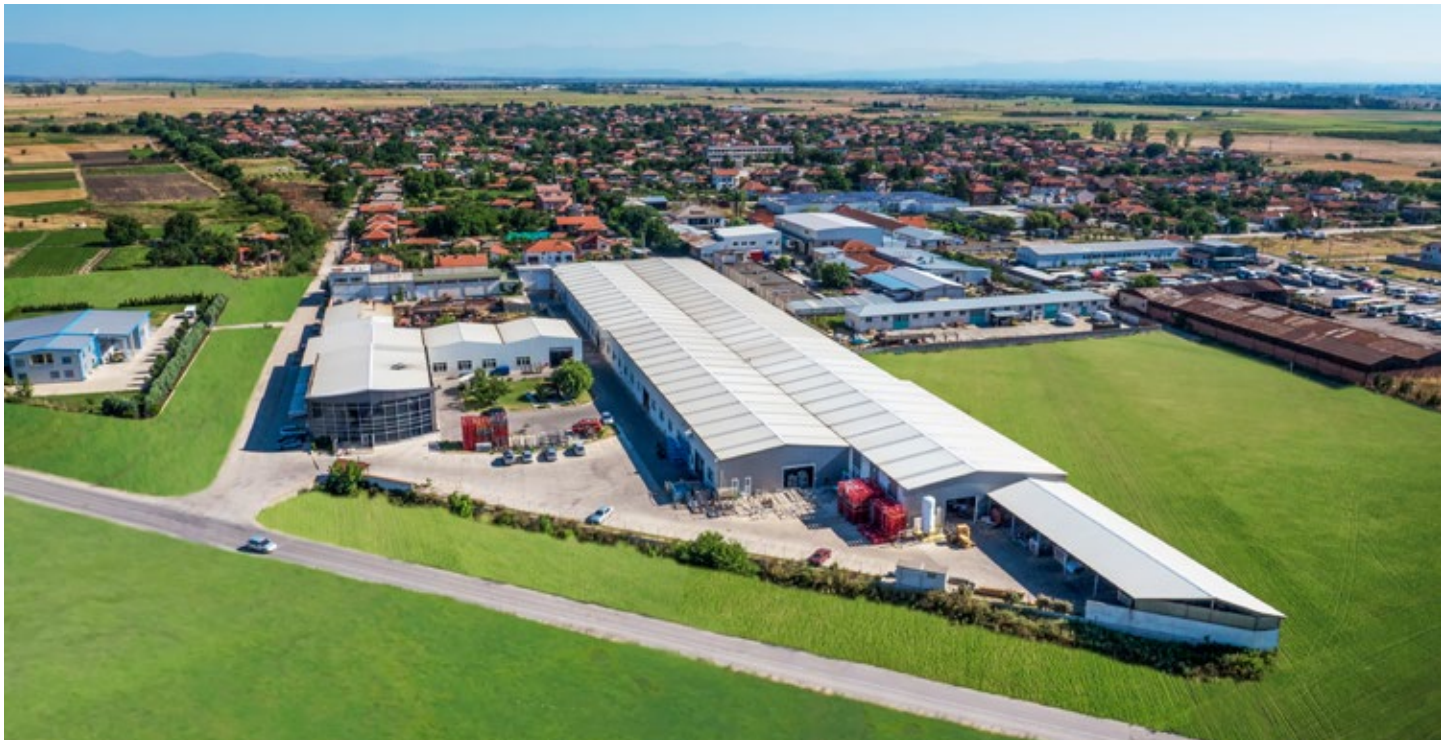
The Marica site is continuing to develop further, and its area of roughly 10,000 m 2 allows plenty of space for future activities.
