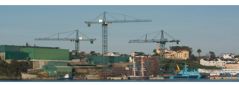
A third Liebherr crane was installed in the Astilleros Gondán, S.A. Castropol (Asturias) shipyard in northern Spain at the start of 2015. After a 1250 HC 50 (since 2009) and a 1250 HC 40 (since 2012) the group has now been supplemented with a new 1900 HC 60. The tower cranes will permanently stretch high into the sky and provide faithful service to the shipbuilding company.
