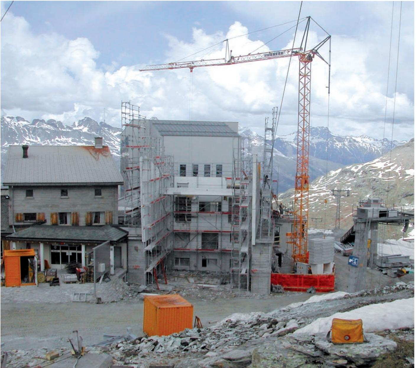
The Murtèl mid-way station on Piz Corvatsch is being extended by the construction company Nicol. Hartmann & Cie. AG at an altitude of more than 2,700 metres, and a Liebherr 34 K fast-erecting crane is hard at work.
