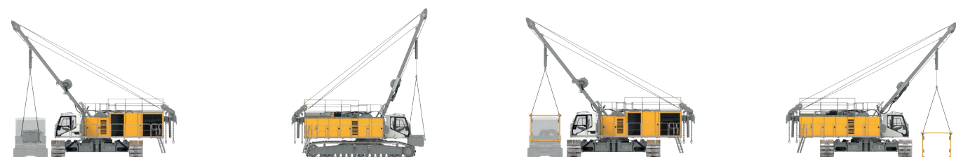
Unloading and assembly of carbody counterweight
